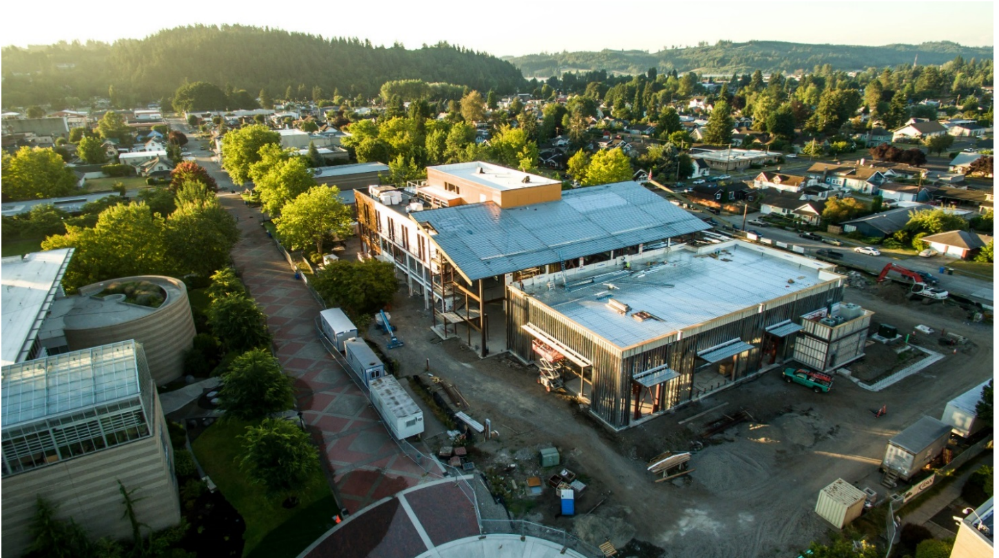
TransAlta Commons Project nearing completion
